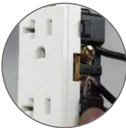
How to Connect Wires to Screw Terminals
