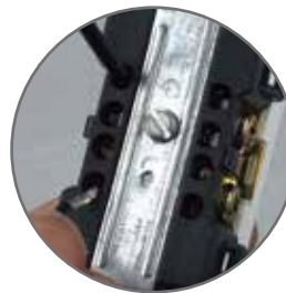
How to Connect Wires with Back Fitting
